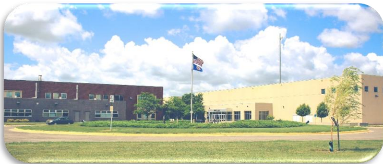
Pipestone Area High School Pipestone, MN
